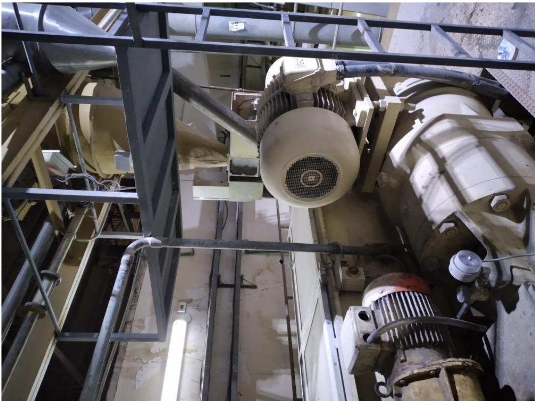
Main Drive and Axial Bearing of Press TPCE
